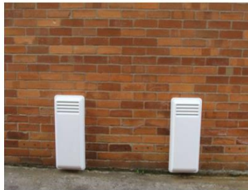
Air Vent Protection
