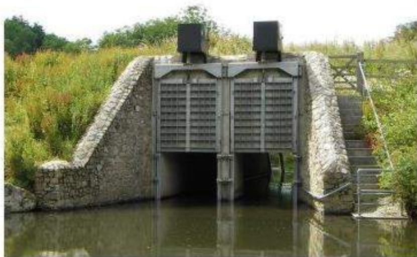
Image of the Palmer's Dam sluice gate
